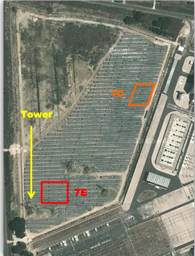
Figure 1: A satellite image of the PV array, with two portions of the array that include Tigo Energy optimizers outlined. The area marked with red, Array 7E, has significant shading due to a large electrical transmission tower. The area marked with orange, which indicates Array 1C, sees minimal shading.
