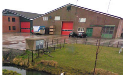
A P. Aker's Flowerbulbs warehouse with cooling rooms.
