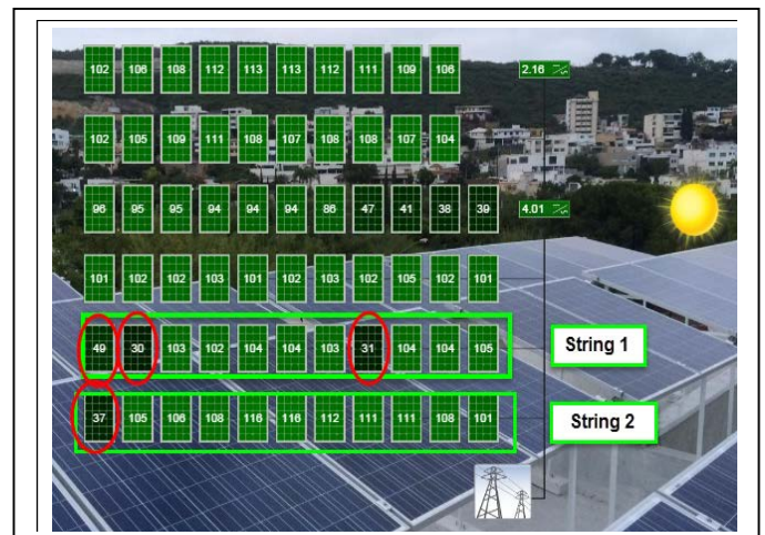
Underperforming panels due to shade do not impact the surrounding modules production.
