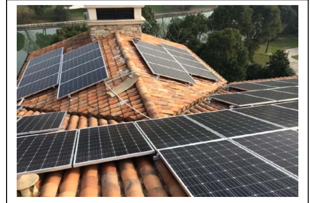
Challenging roof space for panel set up
